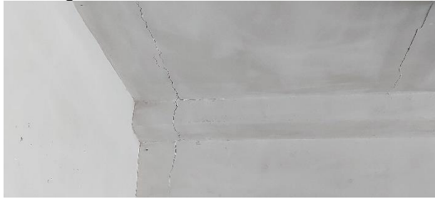
Cracks on the ceiling in the classrooms
